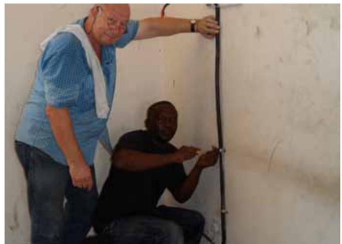
jumped out. Only after installation of the compressor fuse it functioned satisfactorily. During the first pressure expansion we checked the entire compressed air connections and worked at this for leaks.
